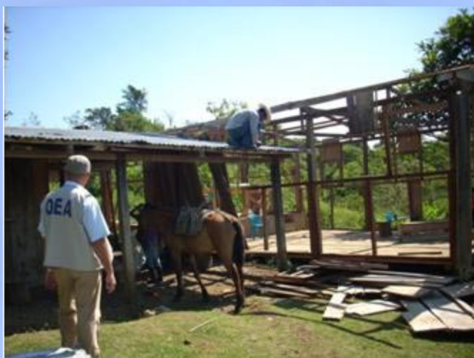
Dismantling of former house
