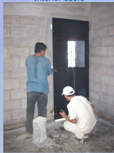
Installing entrance door
