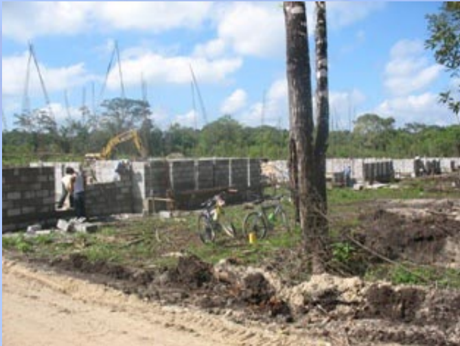
Rear view of construction
