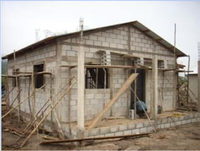
Construction of house in final phase
