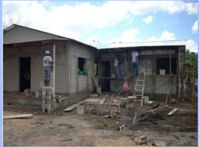
Construction of house in final phase
