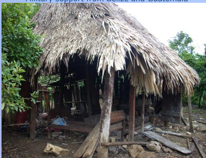
Dismantling of former house
