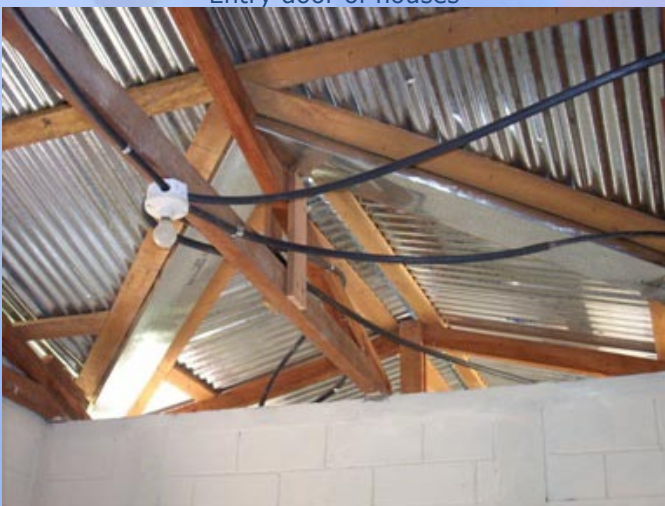
Roofing of houses with electric wiring
