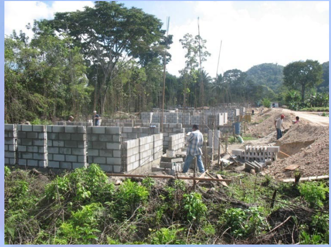
Front view of construction
