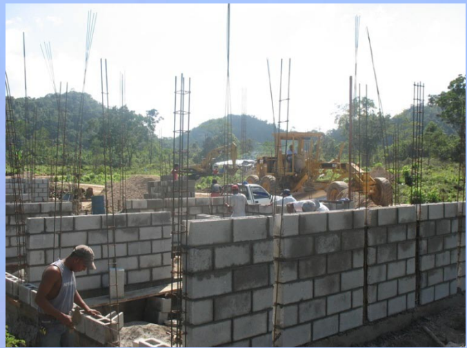
Construction of walls
