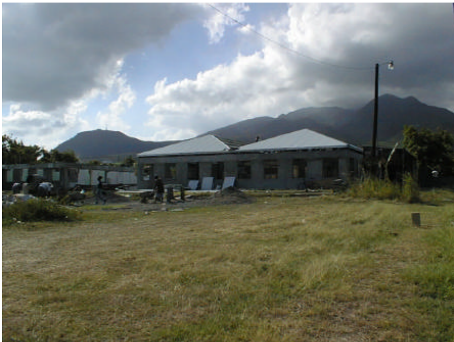
Figure A4-14. J N France Hospital – Strengthened Buildings (St. Kitts)
