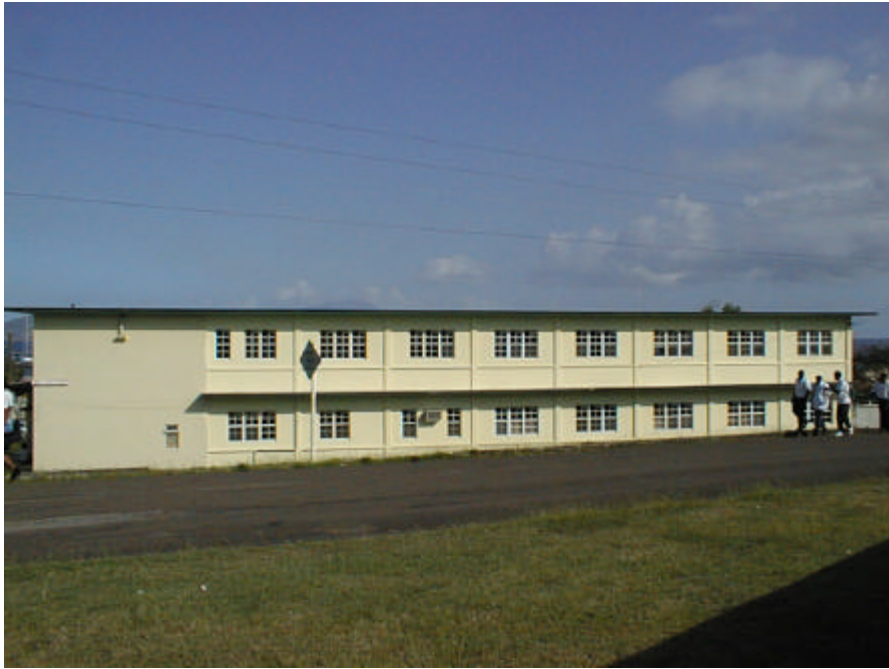
Figure A4-15. Basseterre Health Centre (St. Kitts)
