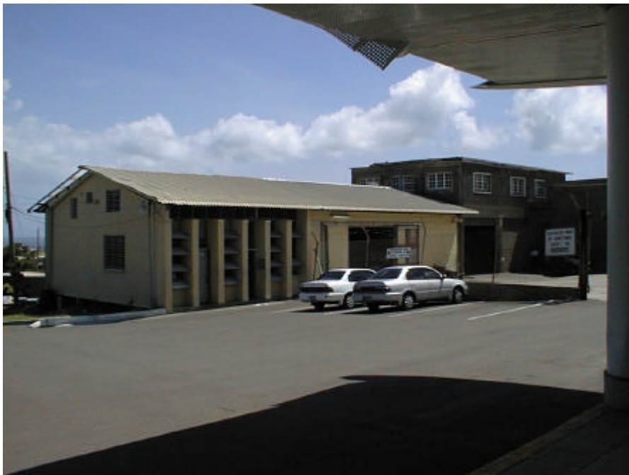
Figure A4-8. Airport Customs Shed (St. Kitts)
