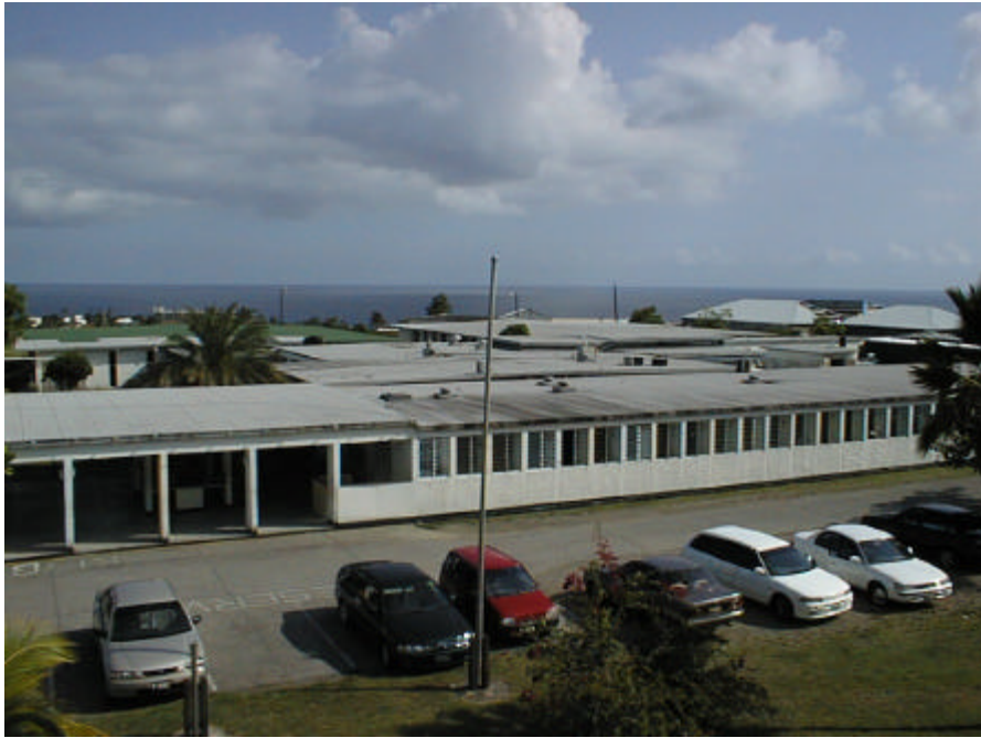
Figure A4-13. J N France Hospital – Existing Construction (St. Kitts)
