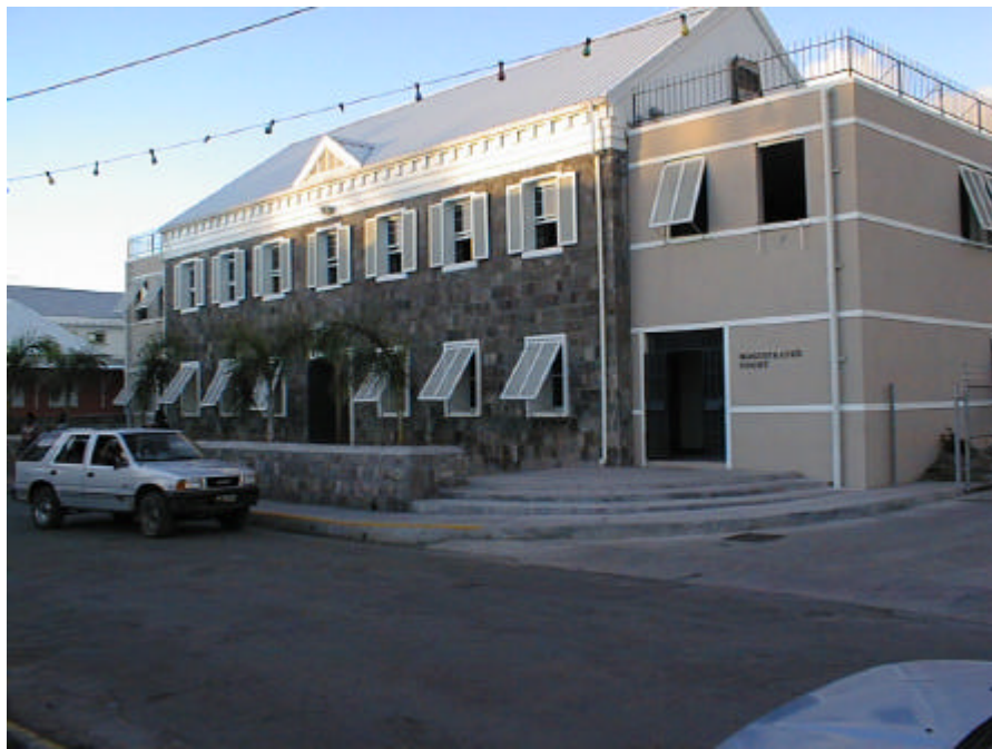
Figure A4-28. Charlestown Police Station (Nevis)
