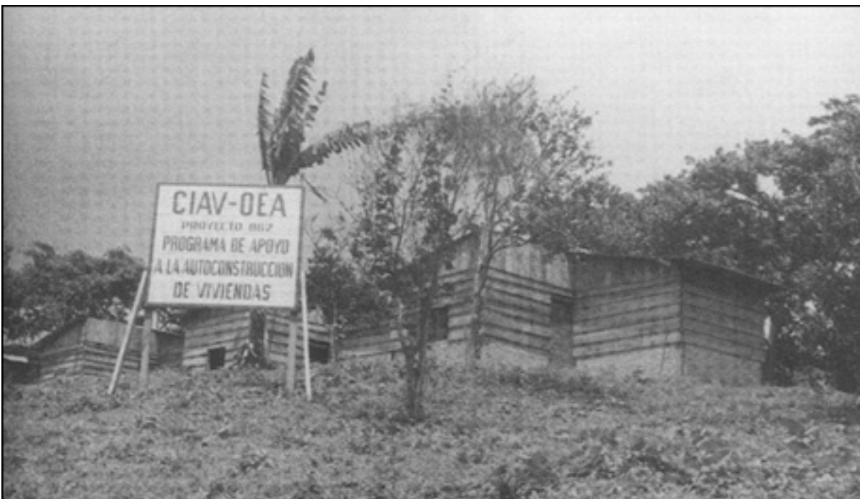
Completed CIAV self-construction housing project in San Rafael del Norte (Nueva Segovia)
