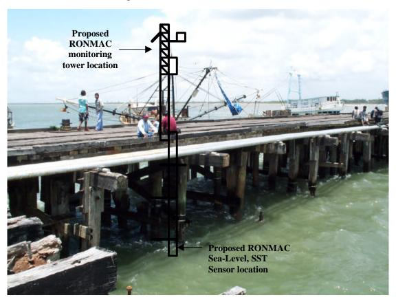
The installation will require "round pile" standoff brackets to compensate for the offset and the slope angle of the pile, however these are the only "good" piles on this side of the pier in an area with sufficient water depth.
