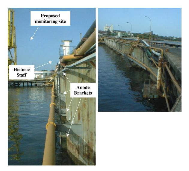
The Proposed RONMAC Monitoring site is located on the extreme edge of the pier roadway, as near to the pier "pipes" as possible. Since the pier is very high above the water, the monitoring site tower is only two sections high and will not require guy wires.
