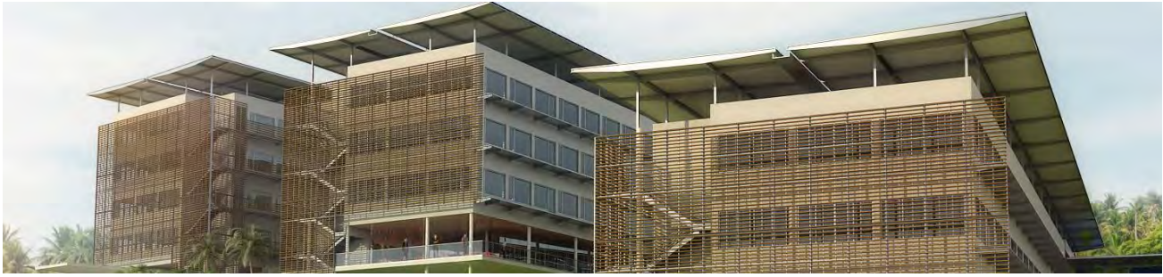
Figure 55- The EE Design incorporates a PV roof protected from extreme winds (top-left). In locations where extreme climatic events are weaker or non-existing, the PV itself can be a solar protection for the façade (top-right, bottom)
