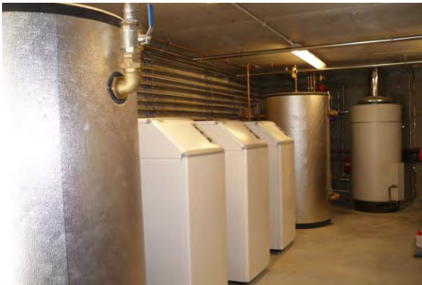
Figure 21-The ground source heat pump, preferably with water (groundwater, seawater etc.) can be placed inside the building and there is no need for cooling towers or external air heat exchangers
