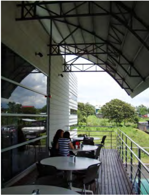
Figure 11- Some constructive elements can be designed to provide solar protection on roofs and façades, protection from the rain and creation of transition spaces (left); protection devices may be fixed or mobile and adapted to the different conditions depending on the orientation
