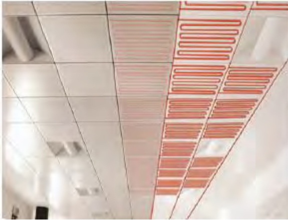
Figure 16-The use of radiant panels on ceilings provides an energy efficient cooling without moving air
