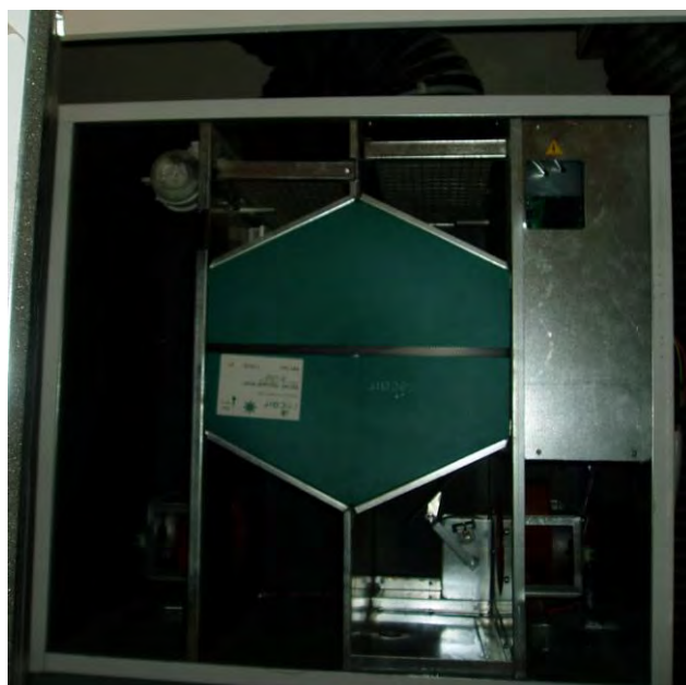
Figure 17- Heat recovery units (heat/cold) reduce the external, fresh and warm renovation air temperature for ventilation
