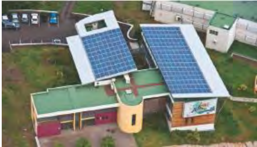
Figure 79- Roof BIPV: Left is North orientation, right, South
