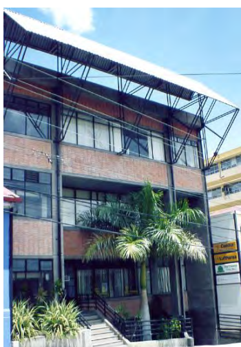
Figure 9- Façades are designed in a different way according to their orientation (left); depending on the latitude the sun path changes is different and thus the incidence on façades and roofs varies. For an average latitude in the Caribbean, the central months of the year represent a considerable incidence on the North façade, as shown by the orthographic projection (right)
