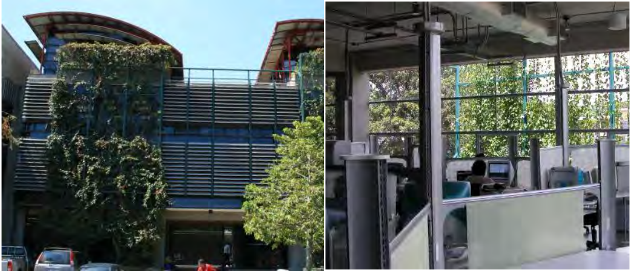
Figure 13-Use of vegetation around buildings reduces the incidence of solar radiation on enclosures, reduces external air temperature and improves the comfort at workspaces
