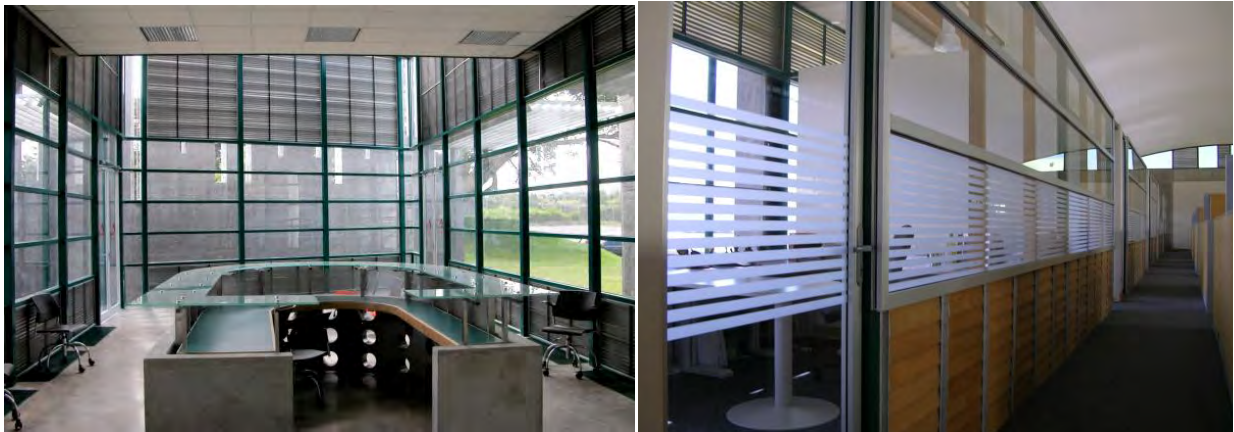
Figure 14-Window-to-wall ratio, the depth of spaces and the use of transparent indoor openings are design criteria that improve daylighting
