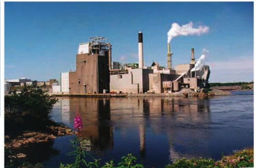
Figure 10. Overview of Irving Pulp and Paper Mill (photo courtesy of Irving)
