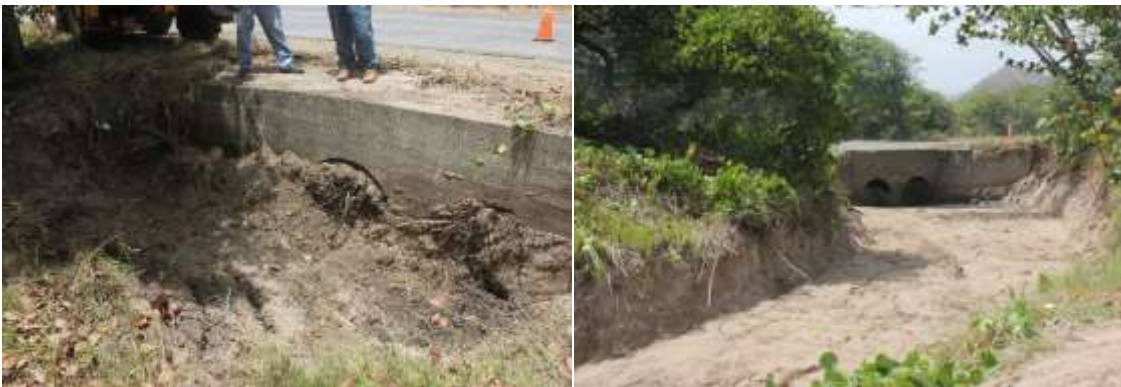
Works in progress on storm water drain clearance
