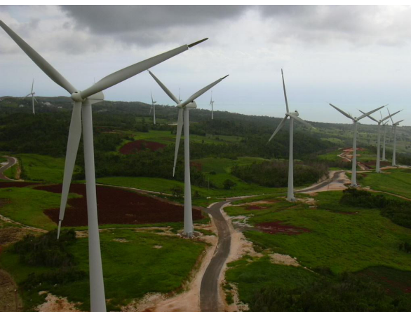
Wind farm located in Wigton, a small rural district in Central Manchester, Jamaica. A similar project in St. Kitts would bring clean renewable energy to the island nation.
