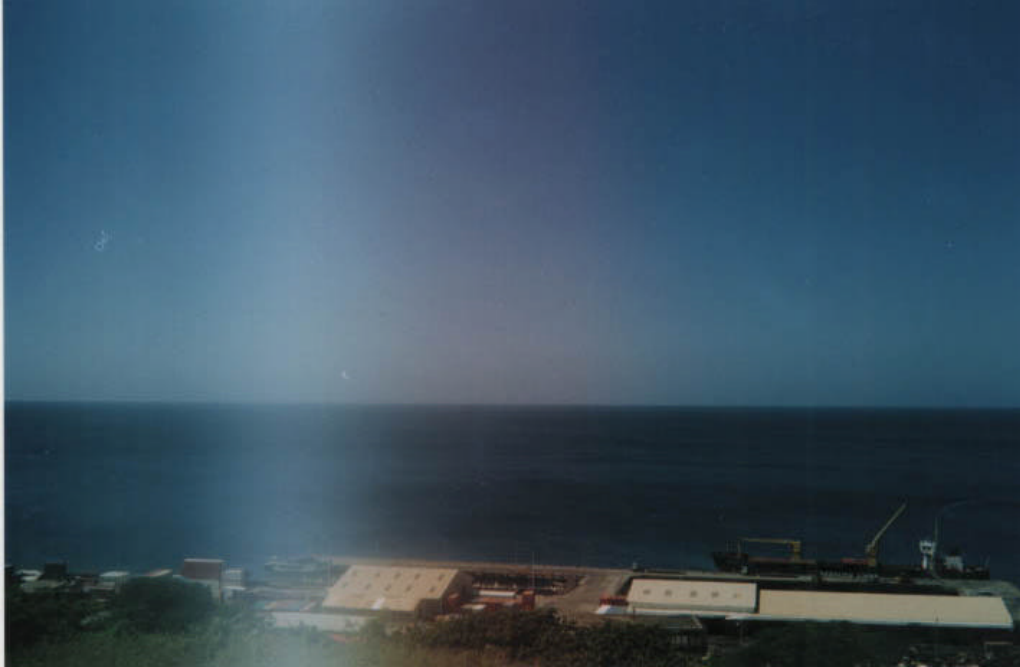
Figure A2-17. Sea Port: Work Frame – Woodbridge Bay (Major Commercial Port, Roseau)
