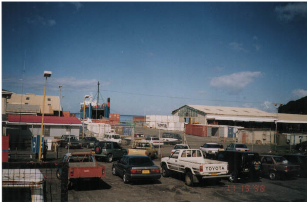
Figure A2-16. Sea Port: Building and Equipment – Major
