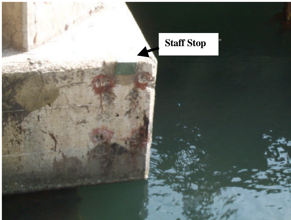
Staff stop (no brackets)
