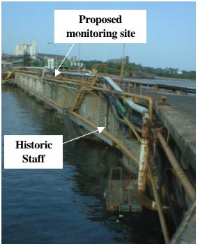
The Proposed RONMAC Monitoring site is located on the extreme edge of the pier roadway, as near to the pier "pipes" as possible. Since the pier is very high above the water, the monitoring site tower is only two sections high and will not require guy wires.
